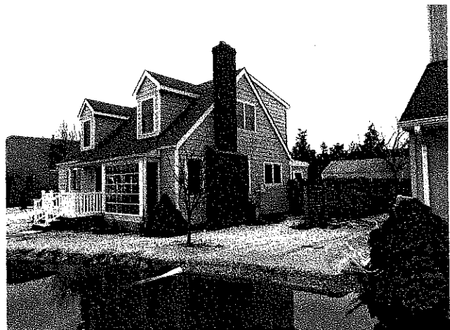
WEST SIDE OF 308 SIXTH AVENUE
