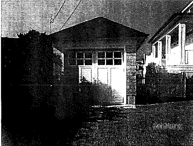
FRONT OF 412 ARROW COURT - DET. GARAGE/CABANA ONLY
