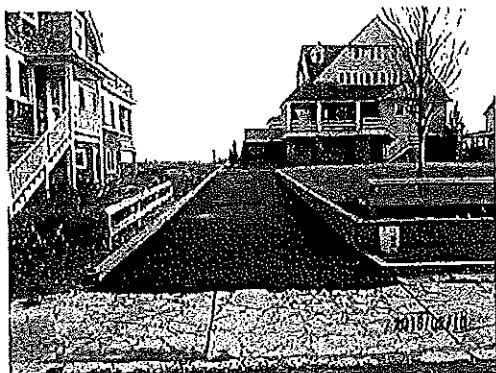
FRONT OF 513 EAST AVENUE
