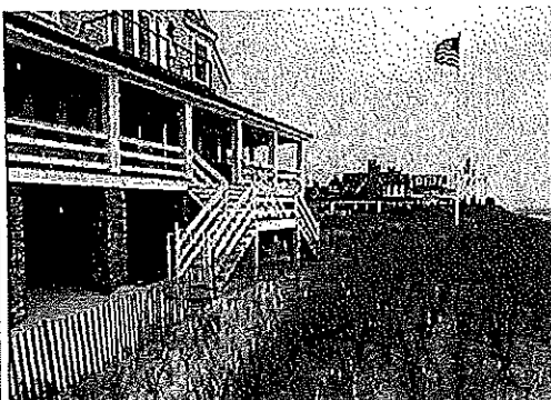
REAR OF 513 EAST AVENUE
