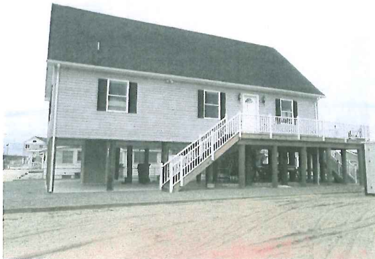
RIGHT SIDE VIEW PHOTO TAKEN 2/10/2015
