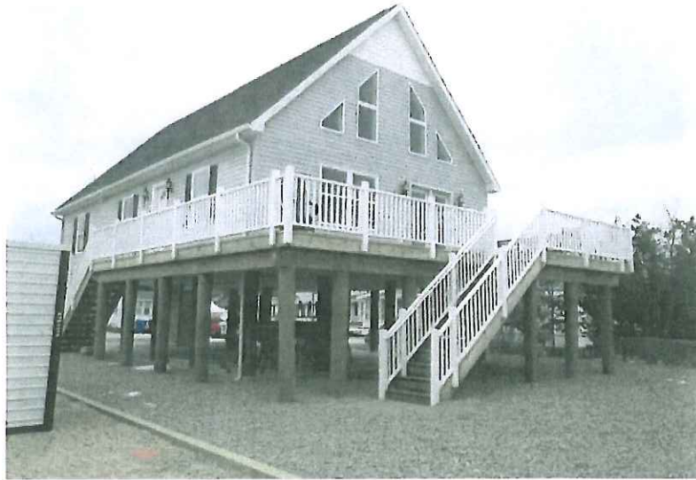
REAR VIEW PHOTO TAKEN 2/10/2015
